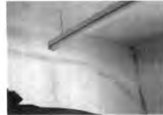
Figure 8: Diagonal crack at the outer edges of concrete framed wall
