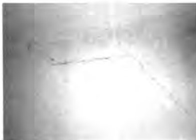
Figure 9: Diagonal crack at the outer edges of load bearing wall
