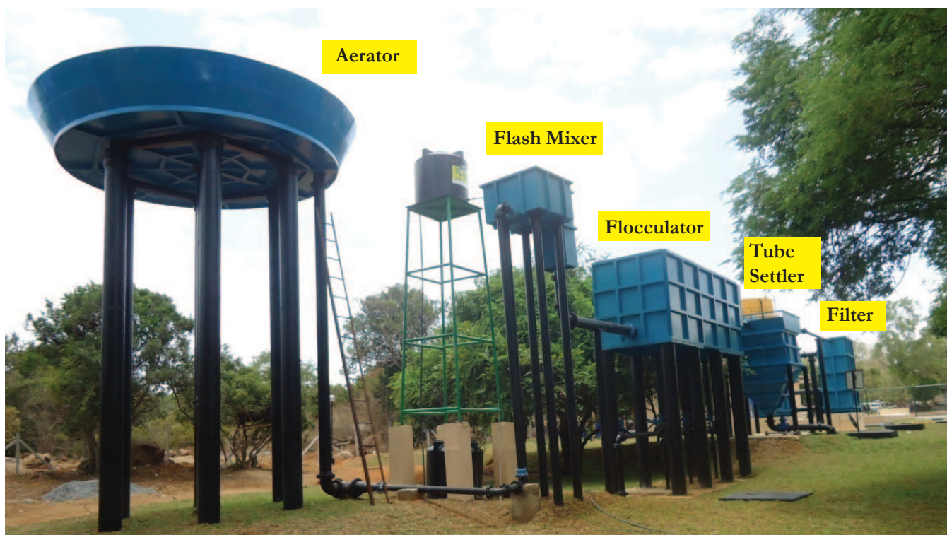
Figure 16 Conventional water treatment plant at Thanthirimale (A joint effort by the Research & Development Unit, the central workshop and the Anuradhapura regional Office of the NWSDB)
