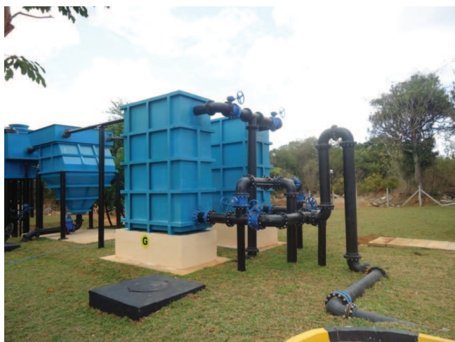
Figure 13 Domestic Slow sand filter (Bio sand filter)
